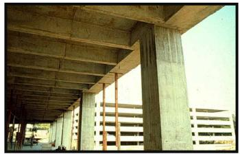
choice, pan joists with wide beams. This system is similar to the filigree system in that the weight of the slab is reduced by introducing voids into them with the pans in order to create ribs. The filigree system might have ended up cheaper since no additional form work is need during construction but structurally the designs should be comparable.
